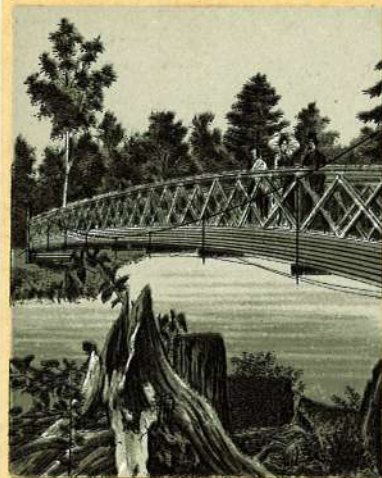
BRIDGE TO SECOND SISTER ISLAND.
