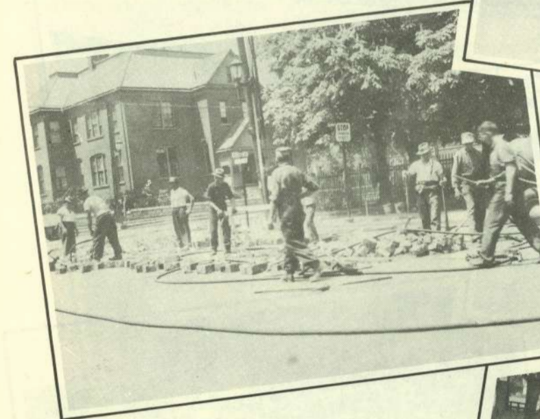
Fig. 4. → Trench completely excavated on one side only, of each rail.
