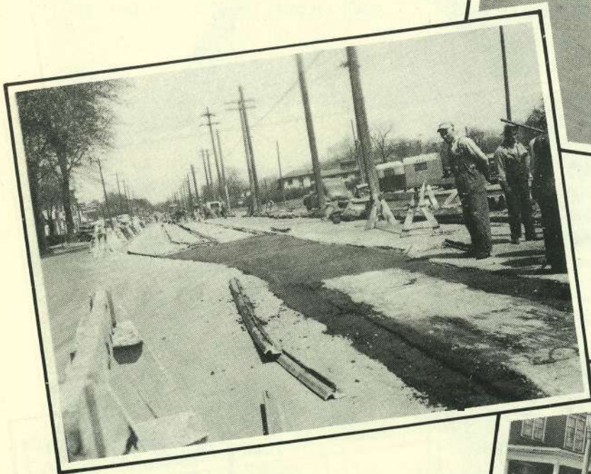
Fig. 22 → Binder course being rolled.
