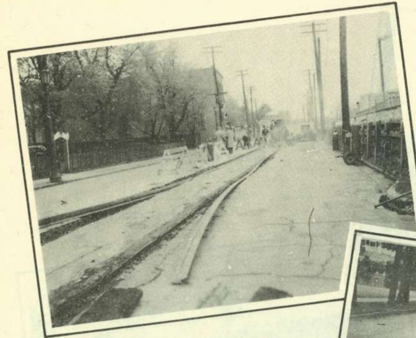
Fig. 18. → General view of burnt rail.
