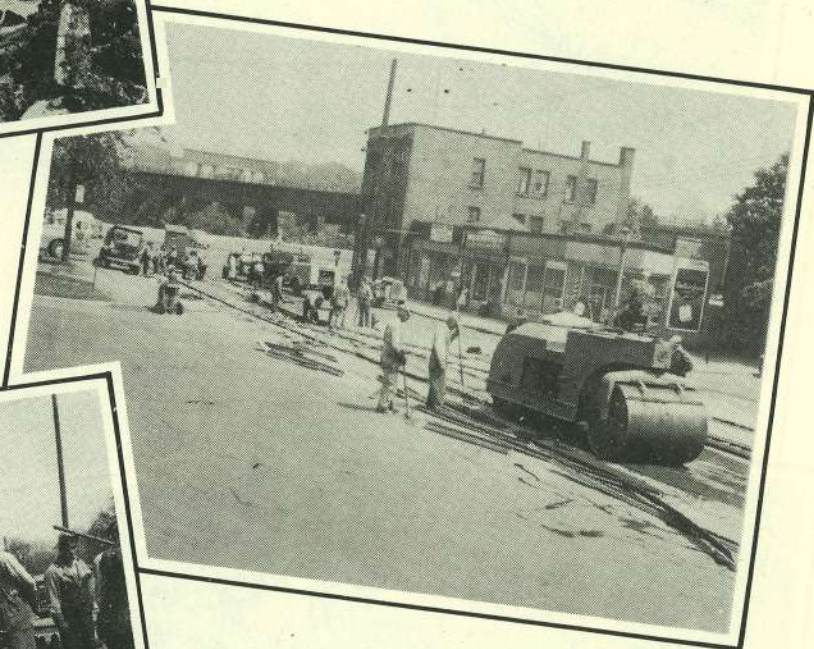
← Fig. 23. Wearing surface in place.
