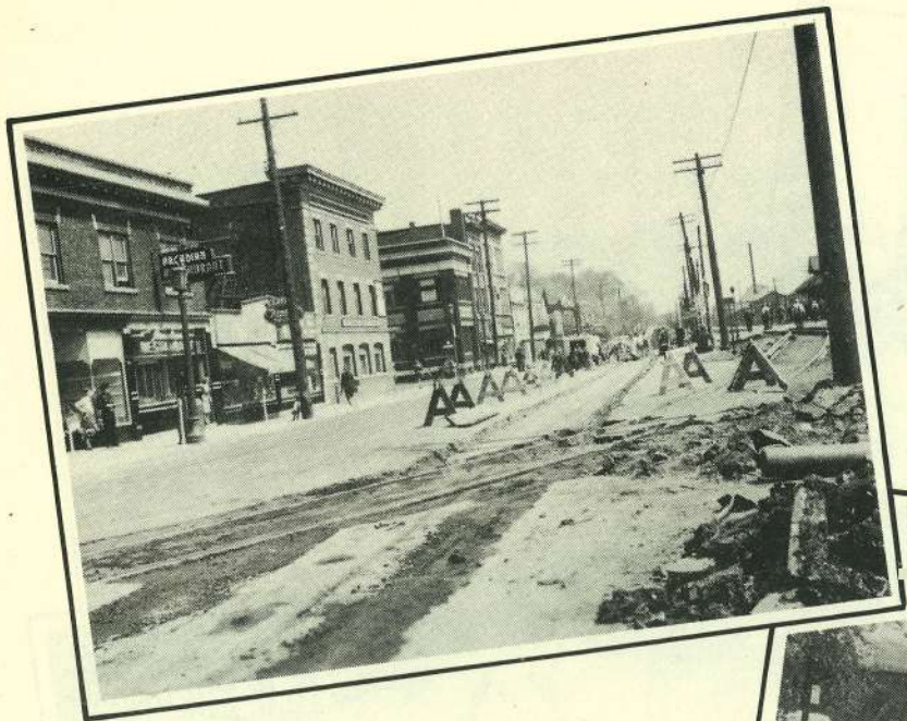
Fig. 22 → Binder course being rolled.
