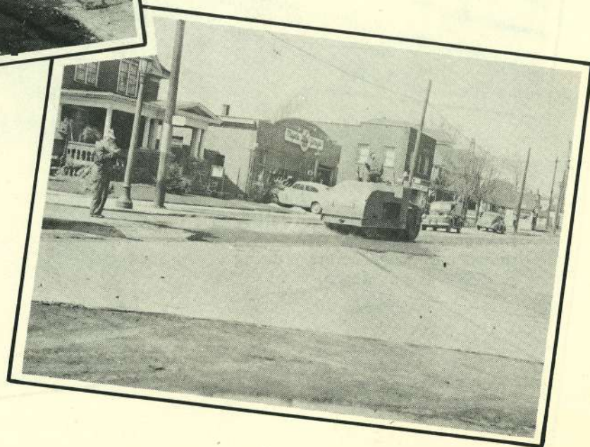
Fig. 24 → Wearing surface being rolled and feathered out to complete paving.
